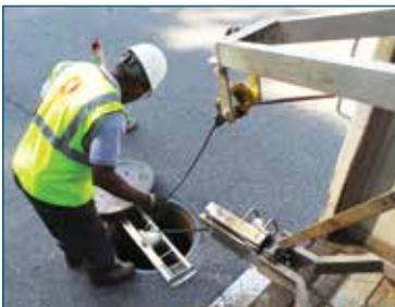
completed from the sewer mainline, but if the inspections cannot be completed from the mainline, inspections are conducted using a push camera, which allows the crew to manually 'push' the CCTV camera from the cleanouts on a person's property to (rather than from) the mainline.
