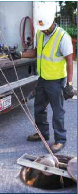
A PEER crew member checks as the CCTV camera enters the sewer via a manhole
